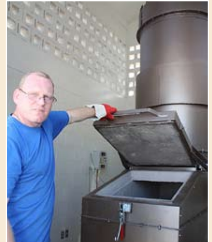
Fired up: The incinerator was installed by the Department of Public Works along with help from a representative of the manufacturer, Inciner8tor, Jason Heaven (pictured).
